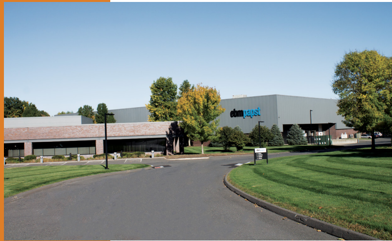
North American headquarters in Farmington, Connecticut
