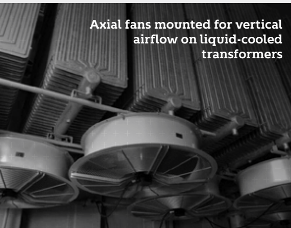
Exhaust face of axial fan for liquid-cooled transformer
